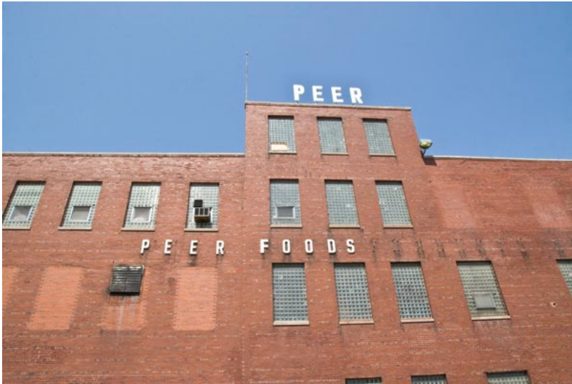
FIG 4.4: The PLANT's home in an ex meat processing facility.
