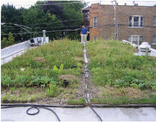
Fig. 3.4.7: Roof after urbanhabitatchicago.com
