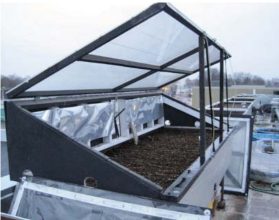
Fig. 3.2.7: Polycarbonate cover on perimeter beds
