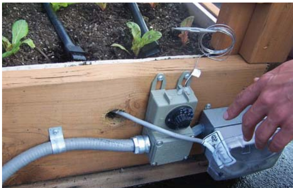
Fig. 3.1.17: Heat cable Willi Galloway, digginfood.com
