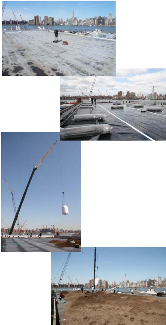
Fig. 3.3.6: Green roof installation series, before, green roof drainage layers, crane lifting medium to roof, medium distribution Lisa Goode
