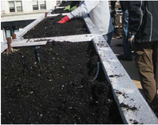
Fig. 3.5.16: Drip irrigation installation Natalie Pfister
