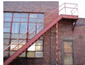
Fig. 3.3.11: Roof access Erin Upton
