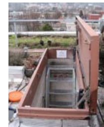
Fig. 3.2.4: The roof hatch
