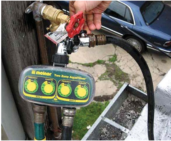
Fig. 3.4.13: Irrigation timer and soaker hose urbanhabitatchicago.com
